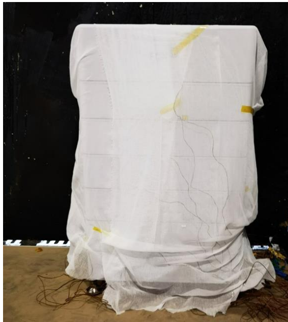
Figure 15: BESS unit after test
